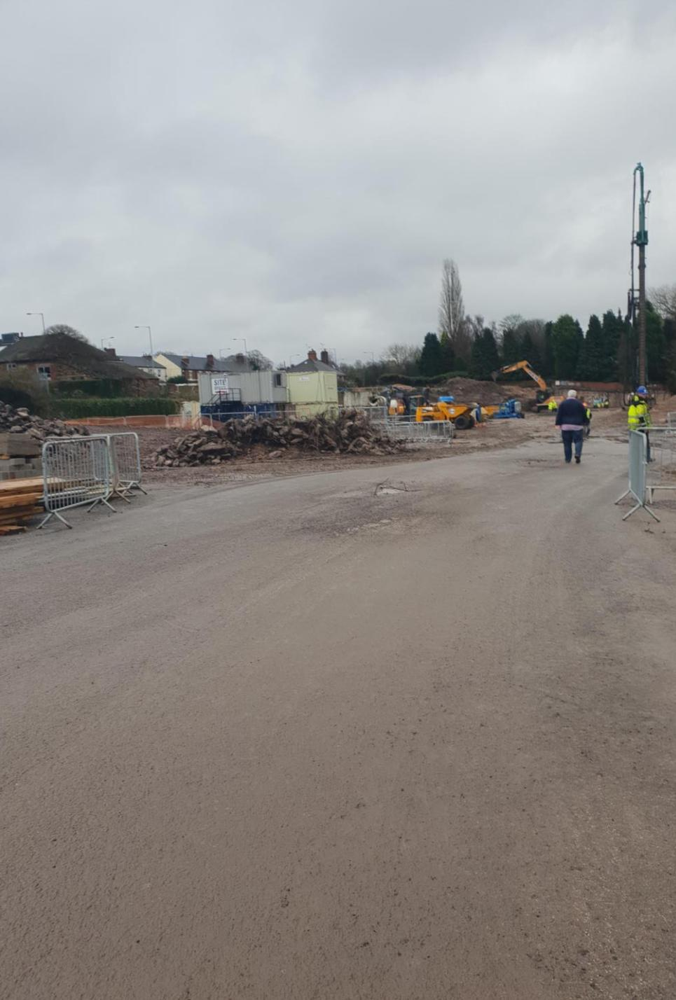
Enabling works commenced in mid-January 2019, ahead of the scheduled commencement date. Initial works have included the establishment of site boundary fencing/hoarding, access and egress routes, removal of underground obstructions/contaminated materials and the breaking up of existing hardstanding areas to allow the material to be crushed and re-cycled.
