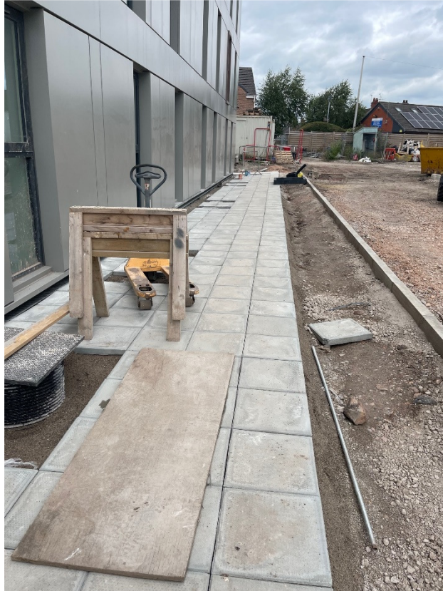
03— Block 04- Paving Installation to Front of Block
